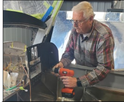
Installing the handsome panel face.
