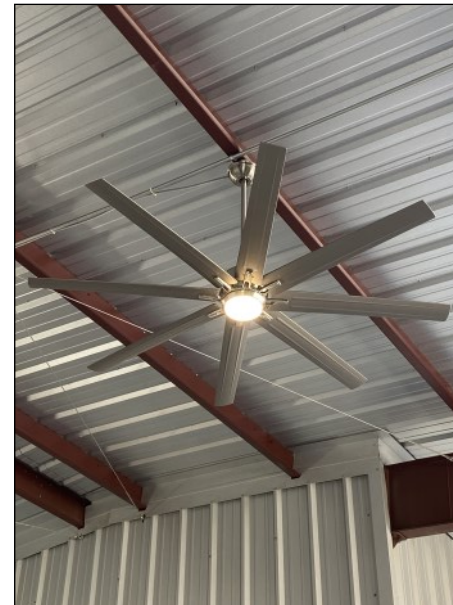
Electrical work—a super fan for improved temperature control, and relocating electrical wiring in preparation for installing the “people door”.
