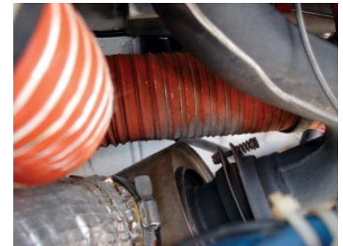
Photo: Evidence of an exhaust leak can be seen on nearby components (photo by Adrian Eichorn)
